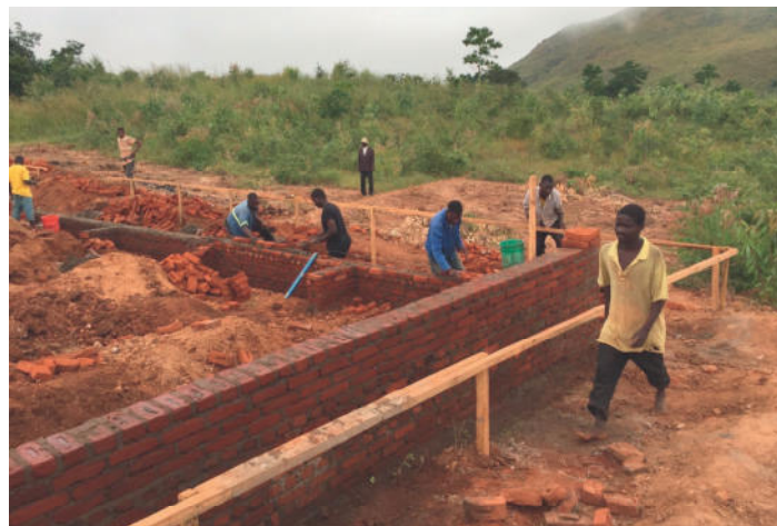
Baustelle in Chikumbu
